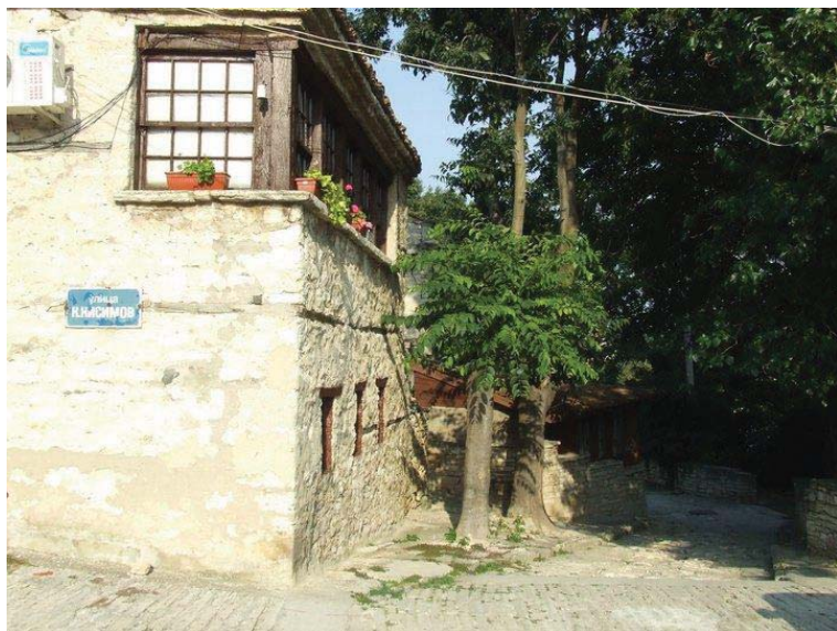
Fig. 87. Vila Ghiul Serai, Balchik (1936), Photo: M. Bostenaru, 2010
