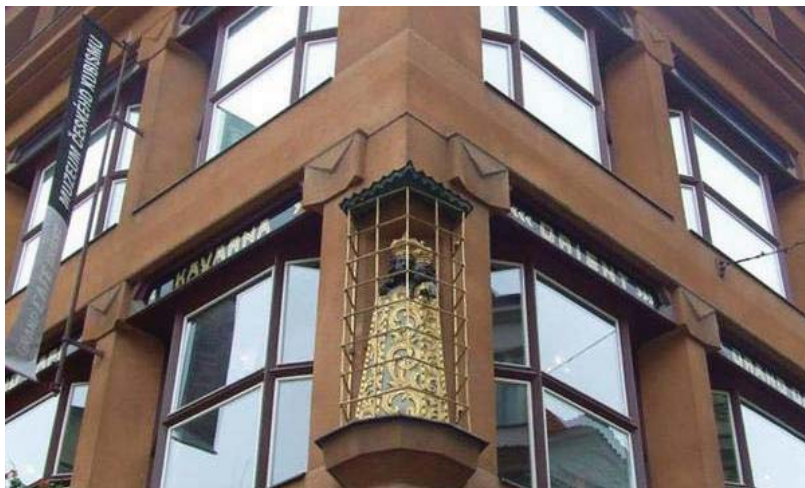
Fig. 28. Czech Cubism. House of the Black Mother of God, Prague. Arch Moskivits Mi-ksa palace, architect Josef Gočár (1911-12) Celetná Str. amd Ovocný trh. Photo: M. Bostenaru, 2008.
