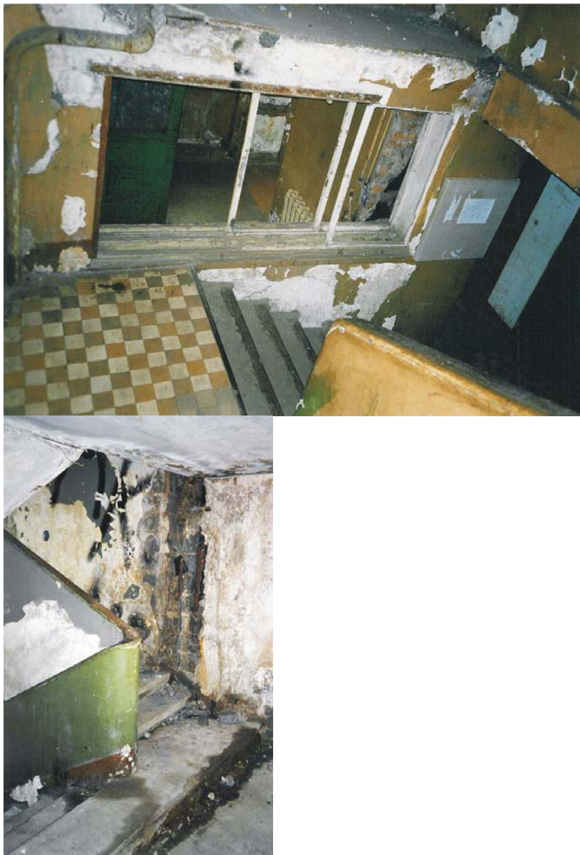
Fig. 60. Narkomfin building, Moscow, architect Moisei Ginzburg with Ignaty Milinis (1928-1932). Photo: Alex Dill.
