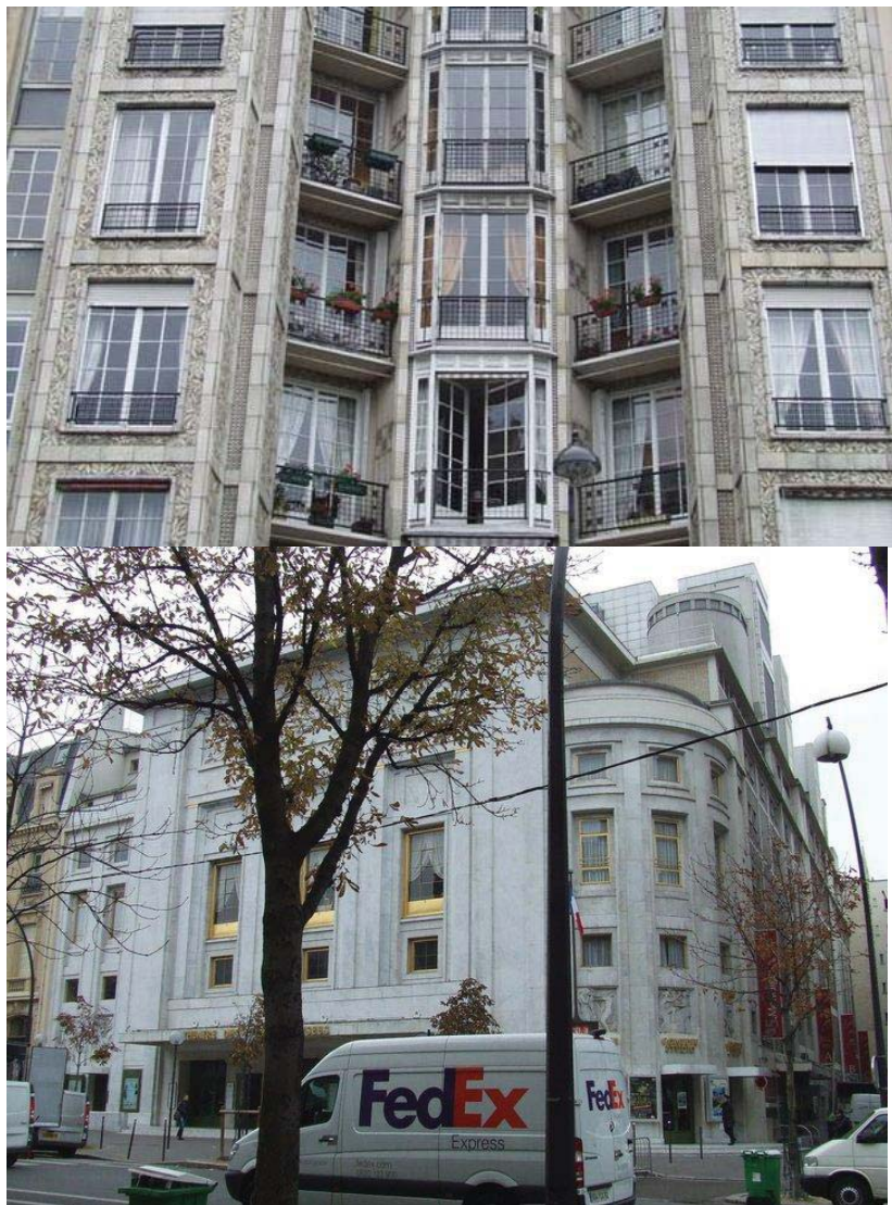
Fig. 25. Architecture of early reinforced concrete in France: Auguste Perret, Paris. Block of flats 25 bis Rue Franklin (1903-1905), Theatre Champs Elysees, 15 Avenue Montaigne (1911-13) (conceived initially by Henri van de Velde). Photo: M. Bostenaru, 2010.
