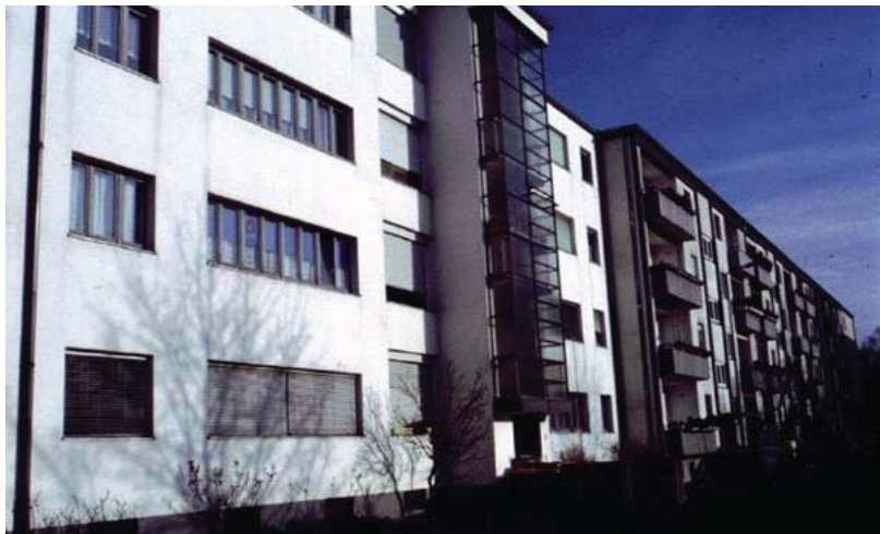
Fig. 26. Interwar architecture with metal skeleton in the Dammerstock Siedlung, Karlsruhe, Germany (arch. Otto Haessler, 1929). Photo: M. Bostenaru, 2002.
