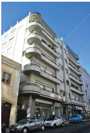
Fig. 65. Building on Rua Nova de São Mamede (1935), Photo: M. Bostenaru, 2013.
