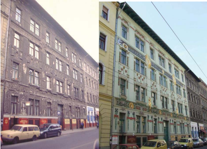
Fig. 138. Block of flats in the Isabella street, Budapest, architect: Frigyes Spiegel (1897), Photos: M. Bostenaru, 2003 and 2006 (before and after restoration).
