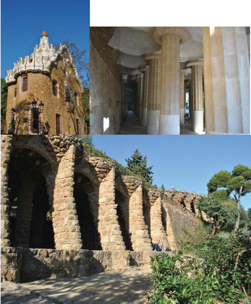
Fig. 24. Parc Güell, arch. Antoni Gaudí (1900-1914). Entrance pavilion, place and viaduct. Photo: M. Bostenaru, 2011.
