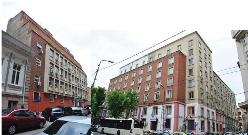
Fig. 85. Gas and Electric Company Building (1945-48), Photo: M. Bostenaru, 2014
