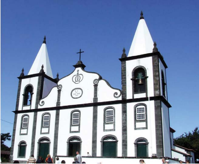
Fig. 68. Combination of white plaster and volcanic stone in a church in the Azores architecture, Photo: M. Bostenaru, 2008
