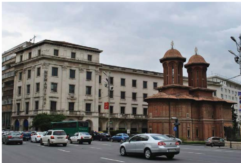
Fig. 83. Corpus of the Kretzulescu Church Wardship (1938), Photo: M. Bostenaru, 2014
