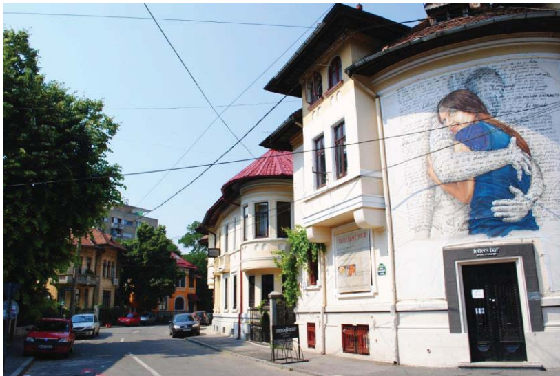
Fig. 131. Group of villas (1929), Photo: M. Bostenaru, 2011
