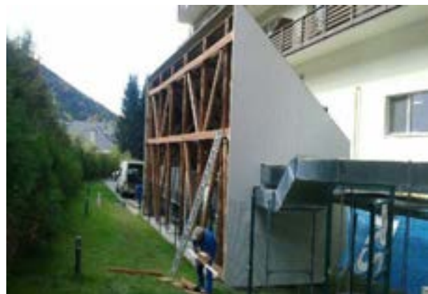
Fig. 5: The minimum height of the screen is determined graphically so that it is below the acoustic shadow line (which joins the highest point of the source with the highest point of the receiver)
