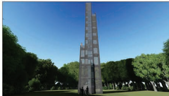
VIEW FROM UNDER THE TOWER
