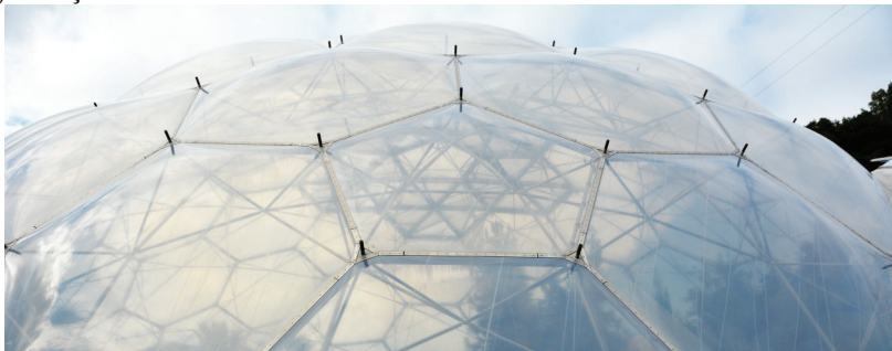
Fig. III.21 – Perne umflate de ETFE, Eden, arhiva arh. Mihai Man
