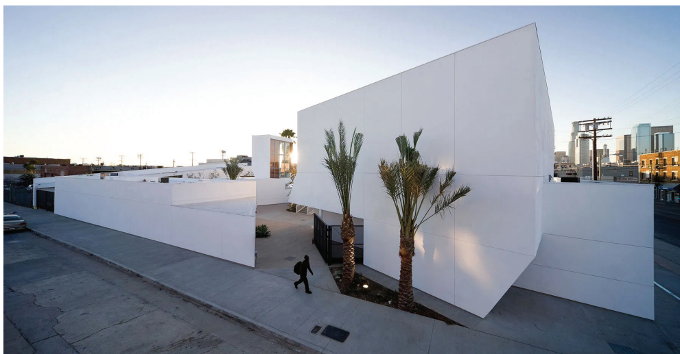
Fig. 5. Inner-City Arts Campus, Los Angeles, SUA – Michael Maltzan Architecture (c) Iwan Baan https://iwan.com/portfolio/michael-maltzan-inner-city-arts-los-angeles
