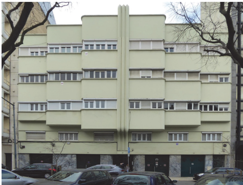
Fig. 266. Imobil de raport, Avenida Defensores de Chaves no. 27, Arh. Cassiano Branco (1937)
