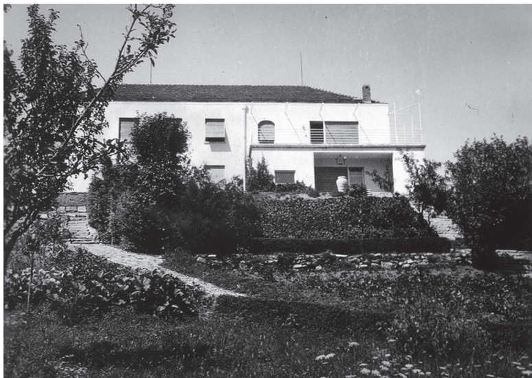
Fig. 8. Villa Tătaru ; Sursa: https://ofhouses.com/post/151781904959/358-elsie-elzy-lazar-gio-ponti-villa
