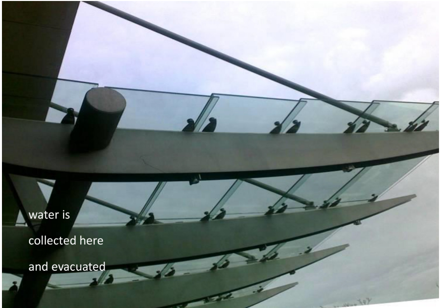
Fig. 5. Glass canopy; water is collected and evacuated.
