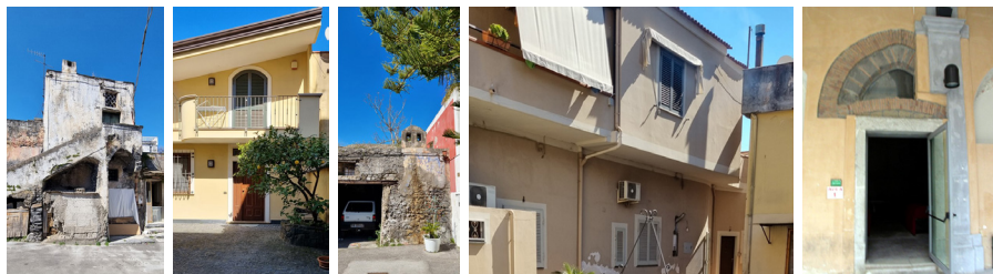
Fig. 13. Buildings – Structural errors. Source: Authors' archive.
