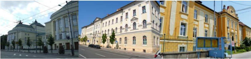
Fig. 3.2: (a) Wivi Lönn Estonia Theater in Tallinn (1913), photo M Bostenaru, (b) Erika Paulas School in Cluj (1902) photo M. Bostenaru (c) Hospital in Medias (1902) photo Alexandru Calcatinge
