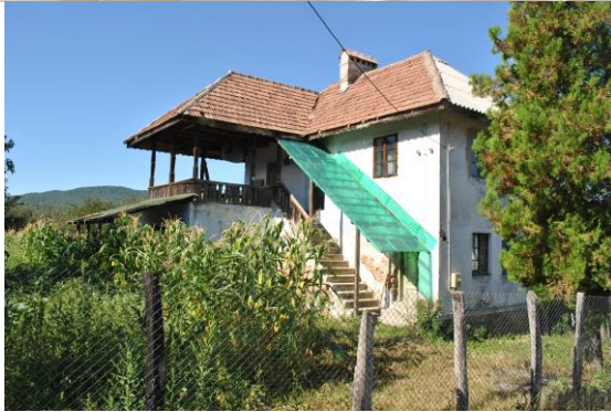
Fig. 4.22: Type F house in the model village of Antonești. Authorization drawings from Pitești county archives, photo: M. Bostenaru.
