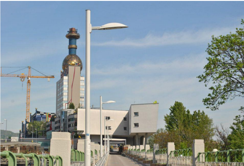
Fig. 4.37: Housing by Zaha Hadid, Spittelau, in Vienna 2005. Photo: M. Bostenaru.
