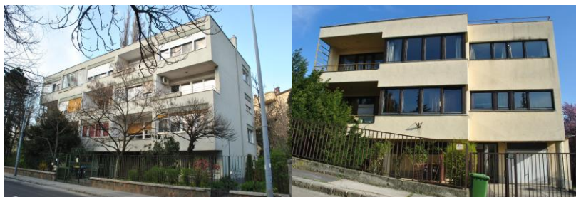
Fig. 2.7: Buildings by Farkas Molnar (second Werkbund) in Budapest, Pasaret neighborhood a neighborhood in Modernist style 1929 Photos: M. Bostenaru.
