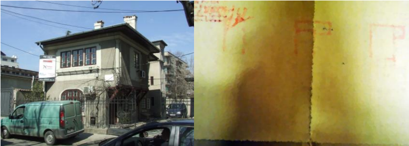
Fig. 4.17: Henriette Delavrancea-Gibory's (1897-1987) own house, built in 1925, Mihai Eminescu Street, Bucharest. Photo: M. Bostenaru, plans, Bucharest municipal archive.
