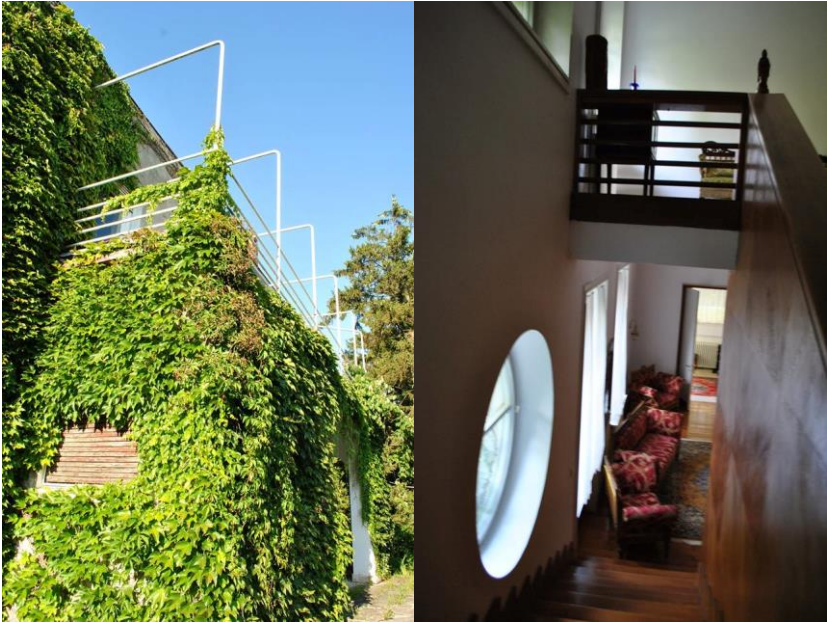
Fig. 3.4: Elsie Lazar Tătaru House, Cluj-Napoca, Romania. Photos: M. Bostenaru.
