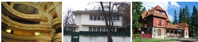
Fig. 4.27: (a) Romanian Youth Palace. (b) Villa Prager, (c) Poiana Țapulului railway station. Photos: M. Bostenaru.
