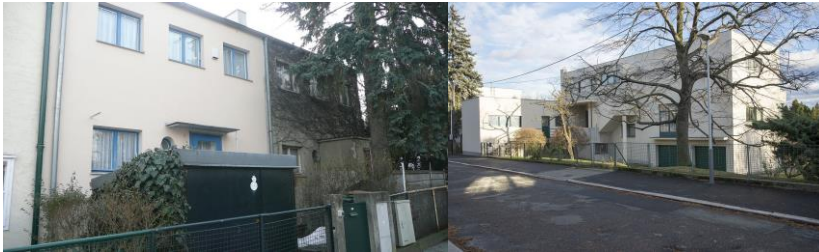
Fig. 2.1: Women architects and Werkbund neighborhoods: (a) Margarete Schütte-Lihotzky, Vienna, 1932, photo wikipedia, (b) Hana Kučerová-Záveská, Czech Republic, Baba Siedlung, Suk House 1932, photo wikipedia.
