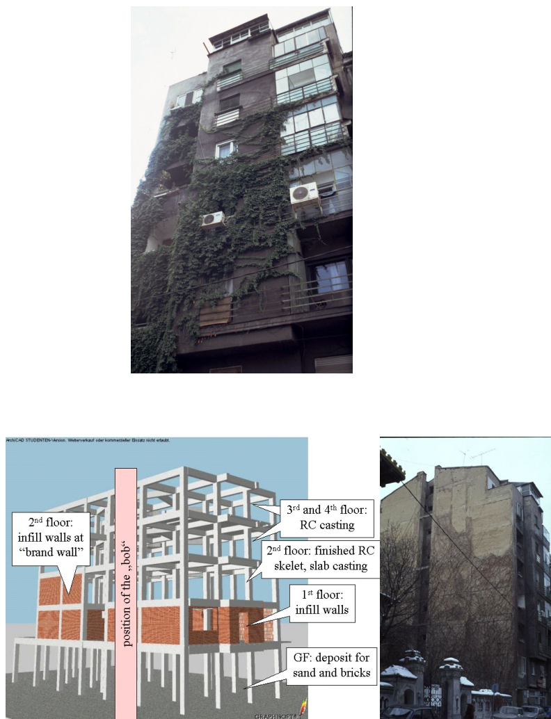
Fig. 100. Naum Ghica building (1938) Schema of the building site organisation for the Naum Ghica building (1938), after Bostenaru (2006), Photo: Maria Boştenaru-Dan, 2002
