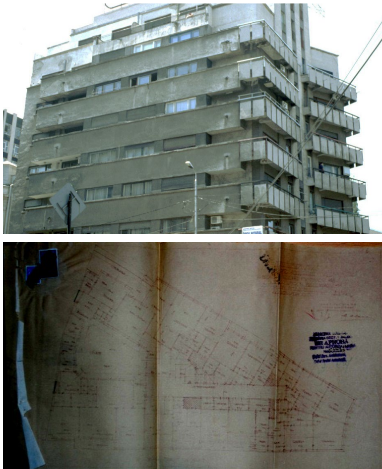
Fig. 6. “Tourist” block of flats (former Palladio, Soc. “Creditul Minier”), architect Marcel Locar (1937). Foto: Maria Boștenaru-Dan, 2002, archive plans: Town hall of Bucharest archives (PMB fond tehnic). Seismic reparation through cutting the corner like in case “Wilson”
